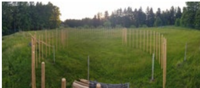
Place of construction and delineation of the building outline on the plot.
